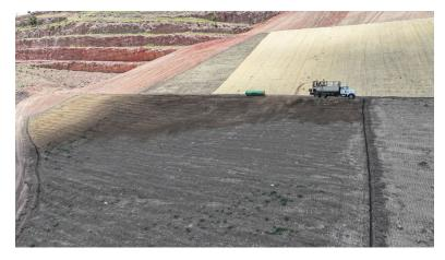
by American Excelsior. Curlex was a critical element of success for the erosion control aspect of the project. Other erosion control products that were used include Profile Products' **ProGanics® DUAL<sup>TM</sup>**, **ProMatrix<sup>TM</sup>**, and **Flexterra®**.
