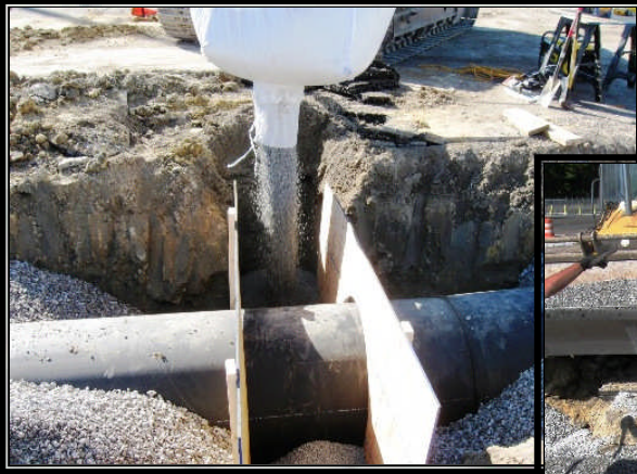
Trench Dam Installations ~ (for sewers and other utilities)
