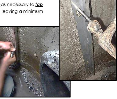
NOTE: If an anchor installation is inadequate, it must be replaced or an additional anchor(s) must be installed on that bracket half.
