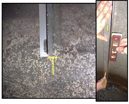
G. Multiple anchor slots are included on each bracket to give the installer options to work around obstructions (e.g. rebar, joint, lift hole). At a minimum, one anchor must be attached at the top and bottom halves of each bracket, and holes must be a minimum of 1.5" deep. Select the desired anchor locations and use a 3/8" concrete drill bit with your drill to make 3" deep holes.
