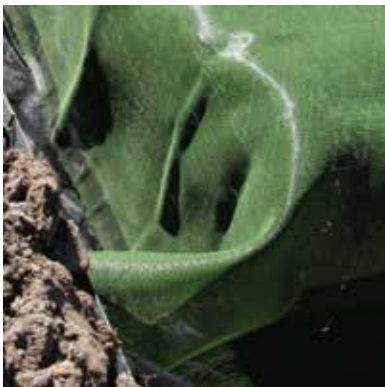
Figure 17: fold corners flat against the tank
