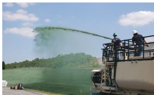
The application of our HydraMax Hydraulic Mulches will work with a wide range of mechanically agitated hydroseeding equipment, and the decreased water-to-mulch mixing ratio will get your job done faster.
