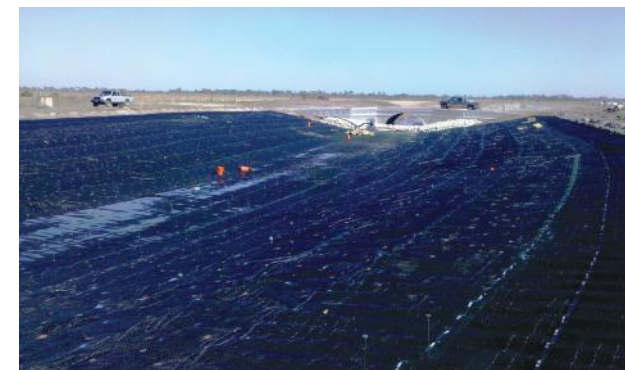
Mary Creek, Archbold Biological Reserve, Central Florida
