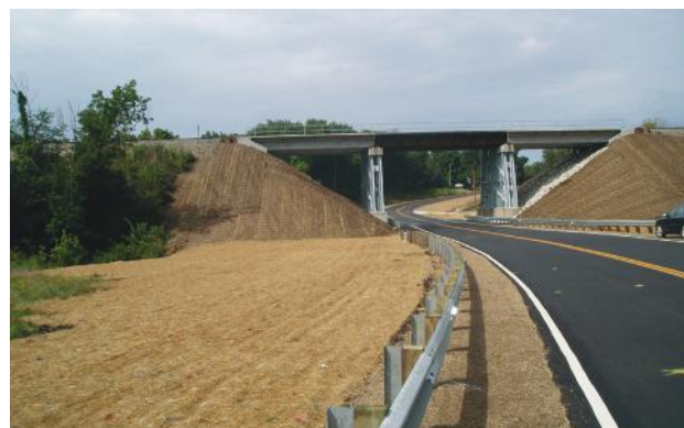
From project start to finish, North American Green erosion and sediment control products will keep you protected until vegetation is established.
