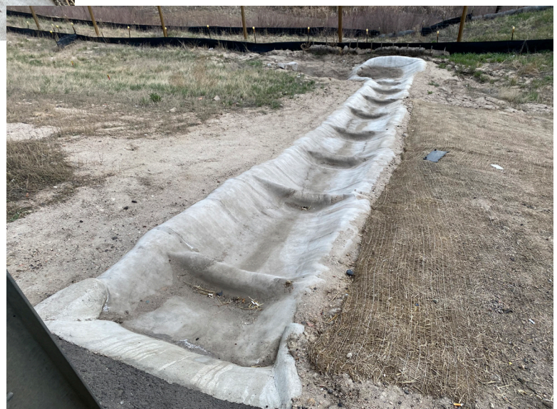
Check Dams & Dissipation Pond Covered in Concrete Canvas
