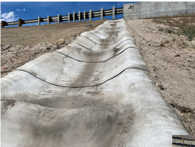
Concrete Canvas Laid Transversely Across the Channel
