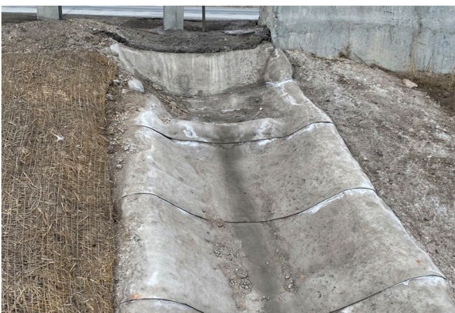
Concrete Canvas Secured with Anchor Trenches
