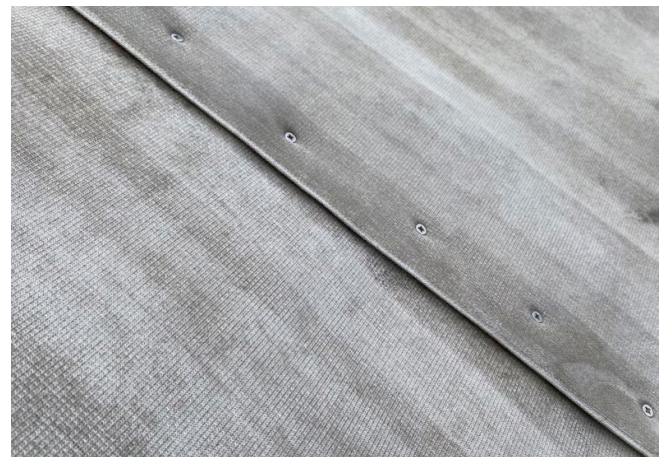
Overlapped CC Layers Secured Using Stainless Steel Screws
