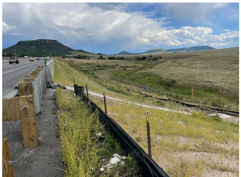
Location of Ditch Next to I-25 Highway
